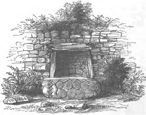
Entrance to Subterranean Chamber.
