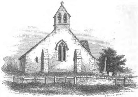
WEST VIEW OF THE CHURCH.
