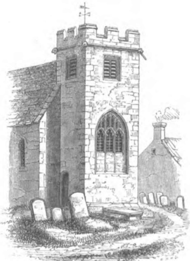
Tower of Cowley Church
