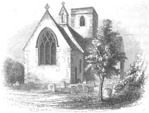
North east view of Church.
